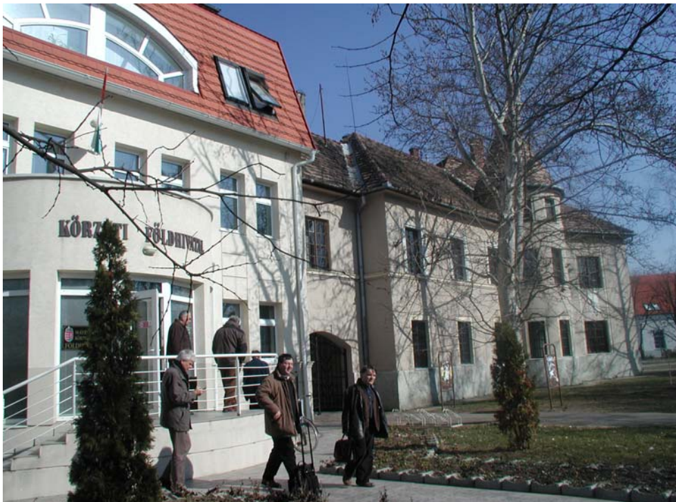
Fig. 3. The building of a District Land Office in the County of Szabolcs-Szatmár-Bereg
