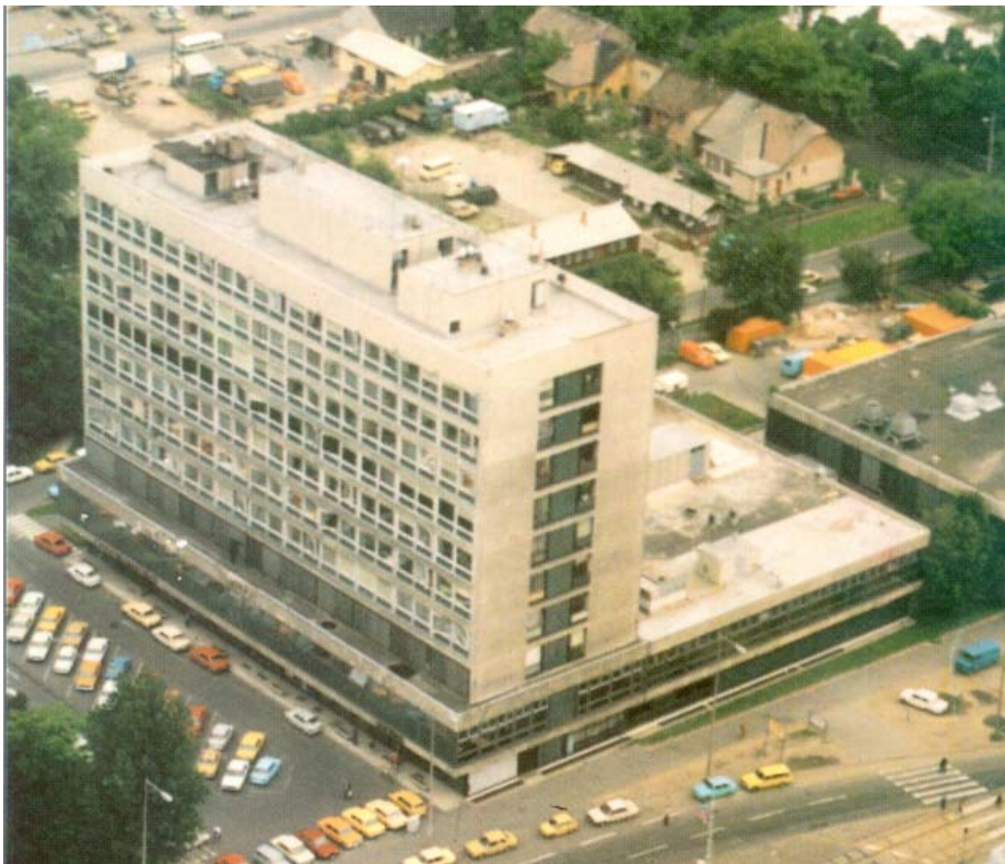
Fig. 2. The building of the Institute of Geodesy, Cartography and Remote Sensing (FÖMI)
